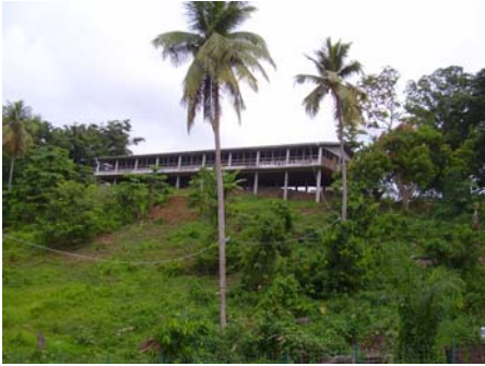
Fig.1 The goat barn. Note the raised floor
