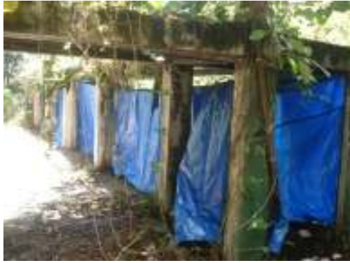
The completed bat tunnel
